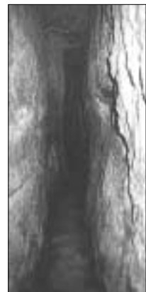
King Hezekiah had this 1,700-foot tunnel chiseled through solid rock to bring the waters of the Gihon Spring from outside the walls of Jerusalem into the city (see 2 Kings 20:20). This reduced the city's chances of being taken by siege—and an Assyrian siege did occur in Hezekiah's time, in 701 B.C. (see 18:13–19:36). In A.D. 1880 an inscription in ancient Hebrew script describing the tunnel's construction was found just inside the tunnel's entrance. Photo: © dlp Studios
